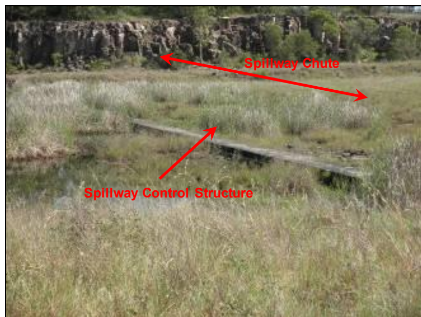
Figure 4: Maroon Dam Spillway.
