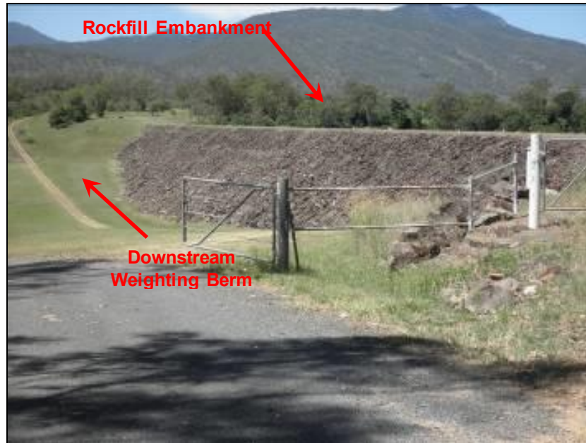
Figure 3: View of Downstream Embankment of Maroon Dam.
