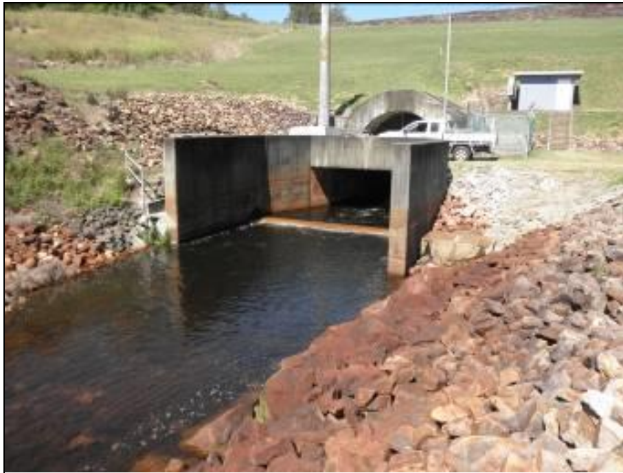
Figure 5: Maroon Dam Outlet – Discharge to Burnett Creek.
