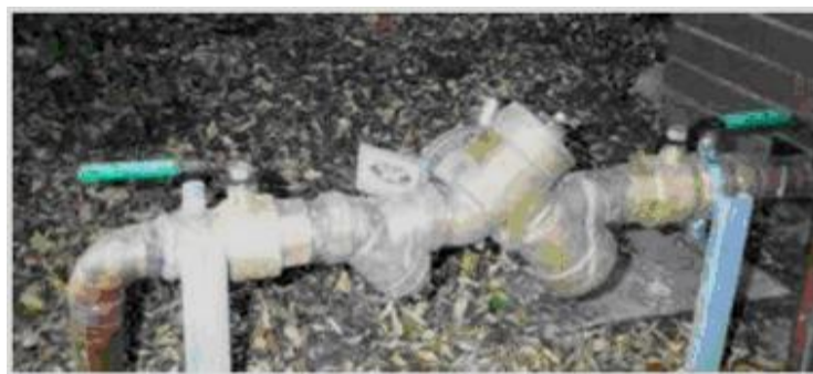
Figure 11: An example of a backflow prevention device. This prevents rainwater being drawn back into the potable mains supply in the event of a pressure drop in the mains water reticulation system.
