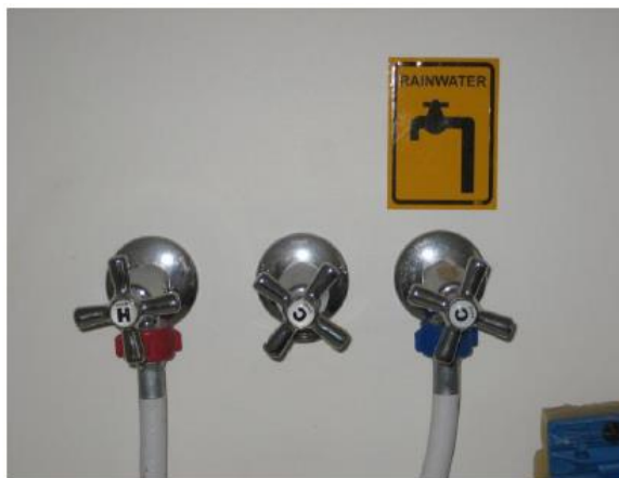
Figure 7: An example of the water supply connection to a washing machine. Note the dedicated rainwater tap as well as mains supplied hot & cold water taps.
