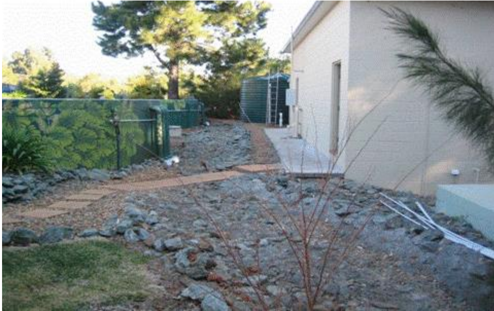
Figure 4: Capo Di Monte wastewater treatment and recycling plant building (external view).
