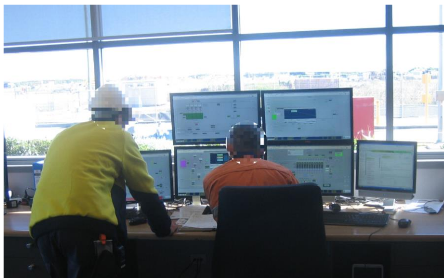
Figure 5: The primary operator console at the AWTP control room. This console is 75-90% attended during shift hours.
