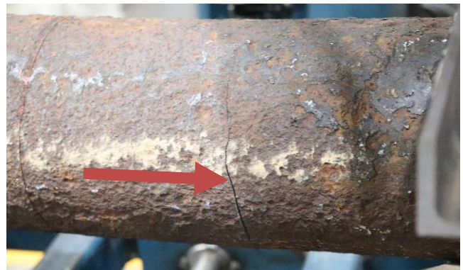
Figure 4: Broken back failure in Trial 3, CI/CL DN125 pipe.
