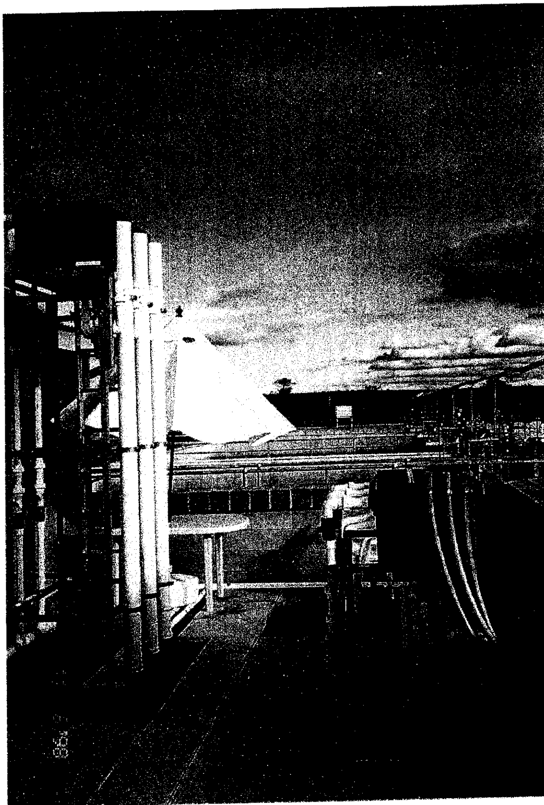
Figure 6.4. Pilot raw water source, chemical addition and mixing at Macarthur WFP.
