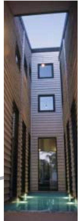
reflection pond at the entrance acts as a passive cooling system throughout the warmer months.
