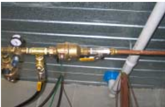
individual meters provide actual rainwater usage per townhouse
