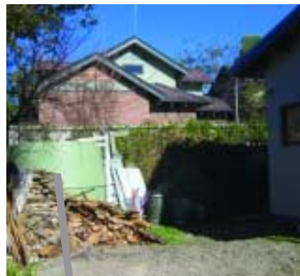
Tank located in unused south east corner of block
