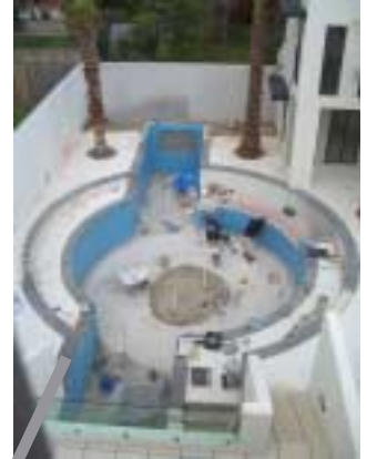
view of pool from rooftop staircase
