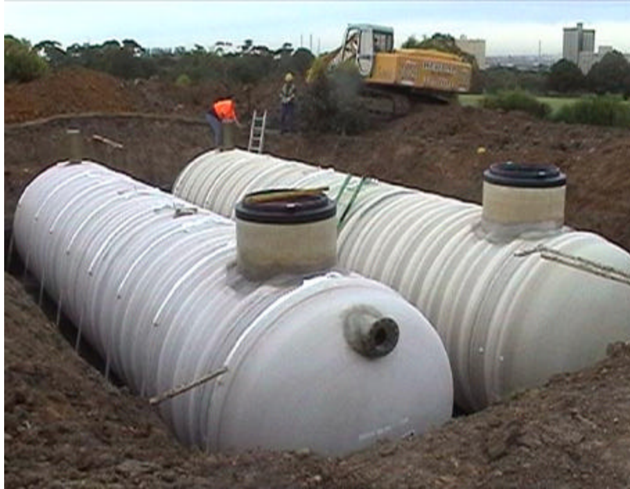
Figure 3 Storage Tanks prior to backfilling.
