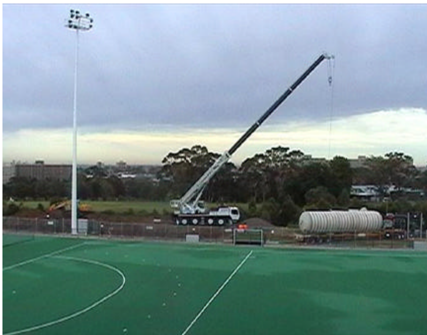
Figure 2 Installation of Storage tanks
