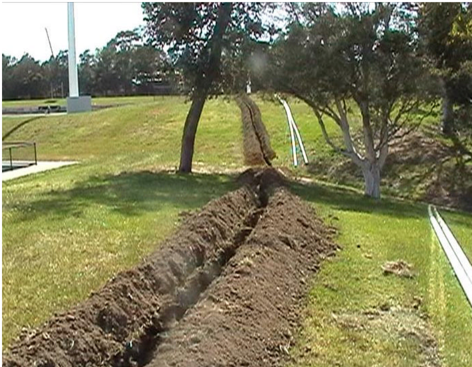
Figure 4 Installation of pipe network
