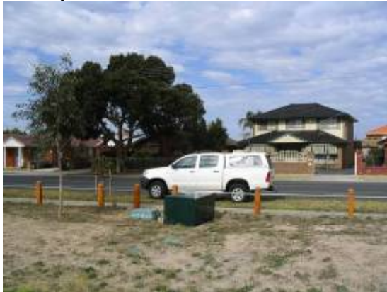
Water meters and potable back up
