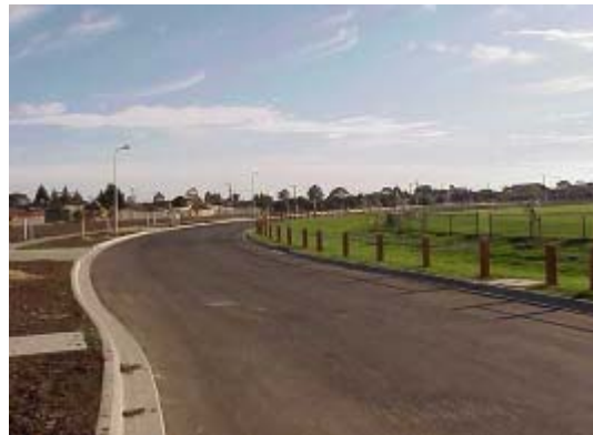
Catchment and grass swale
