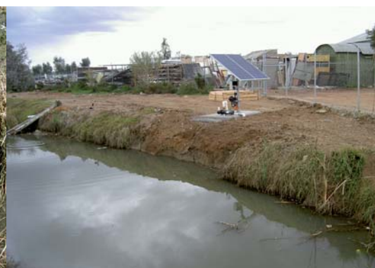
Open drain after excavation
