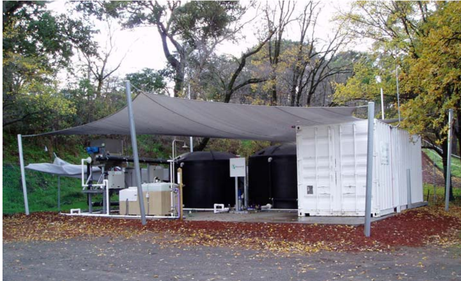
Figure 1 “Flemington Racecourse MWR Demonstration Plant”
