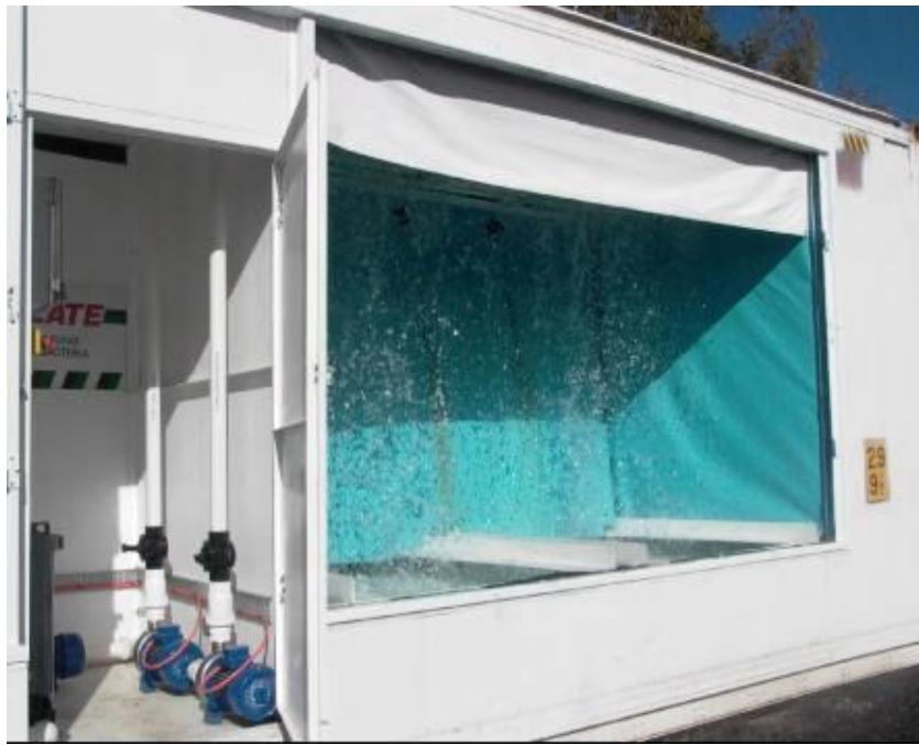
Figure 3.2. Cooling bay 3 and a small plant room of the Smart Water hydrocooler is fabricated from a refrigerated shipping container. The two blue coloured Ebara DWO 400 pumps each extract water from the holding tank of bay 3 and pump it to the water distribution system located in the roof of the shipping container. The water subsequently flows through the produce being cooled. It can be seen that the pipelines leading from the pumps to the water tanks are each fitted with manually operated valves.
