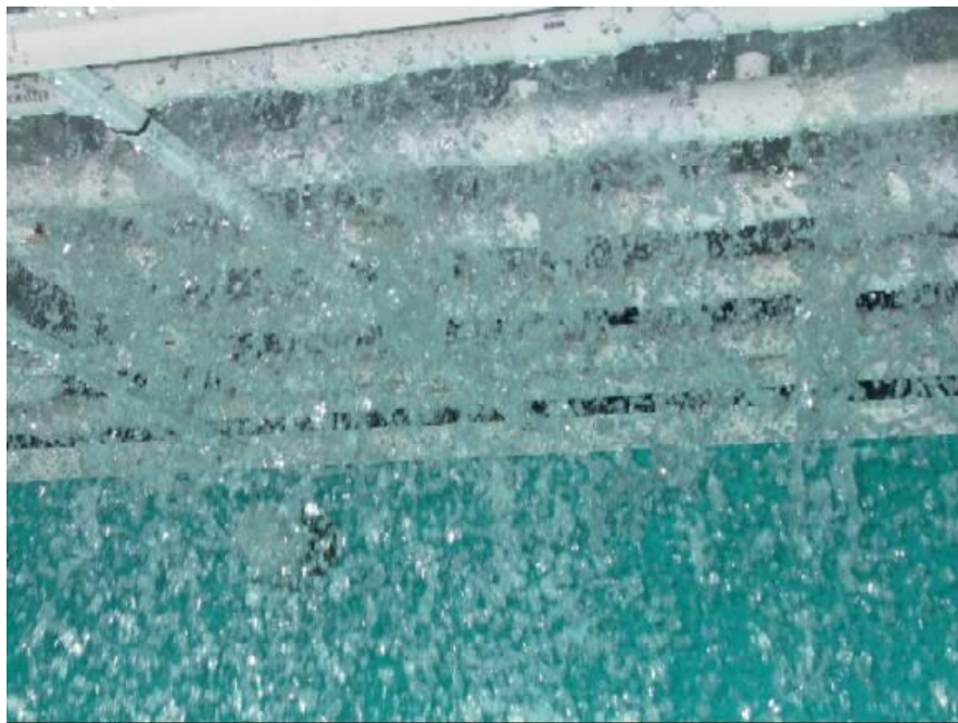
Figure 3.7. Water leaving the distribution system at a rate of about 18 litres per second.
