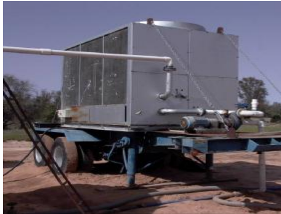
Figure 5.2. The transportable water chilling unit that is used in conjunction with the Smart Water hydrocooler. It is located on a trailer and the pipe leading towards the left of the photograph carries cooled water to the storage tank(s).
