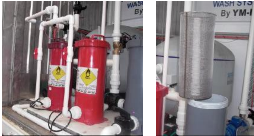
Figure 3.12. The chemical dispensing units (left) and a stainless steel strainer (right). The sand filter is seen in the background of each photograph.
