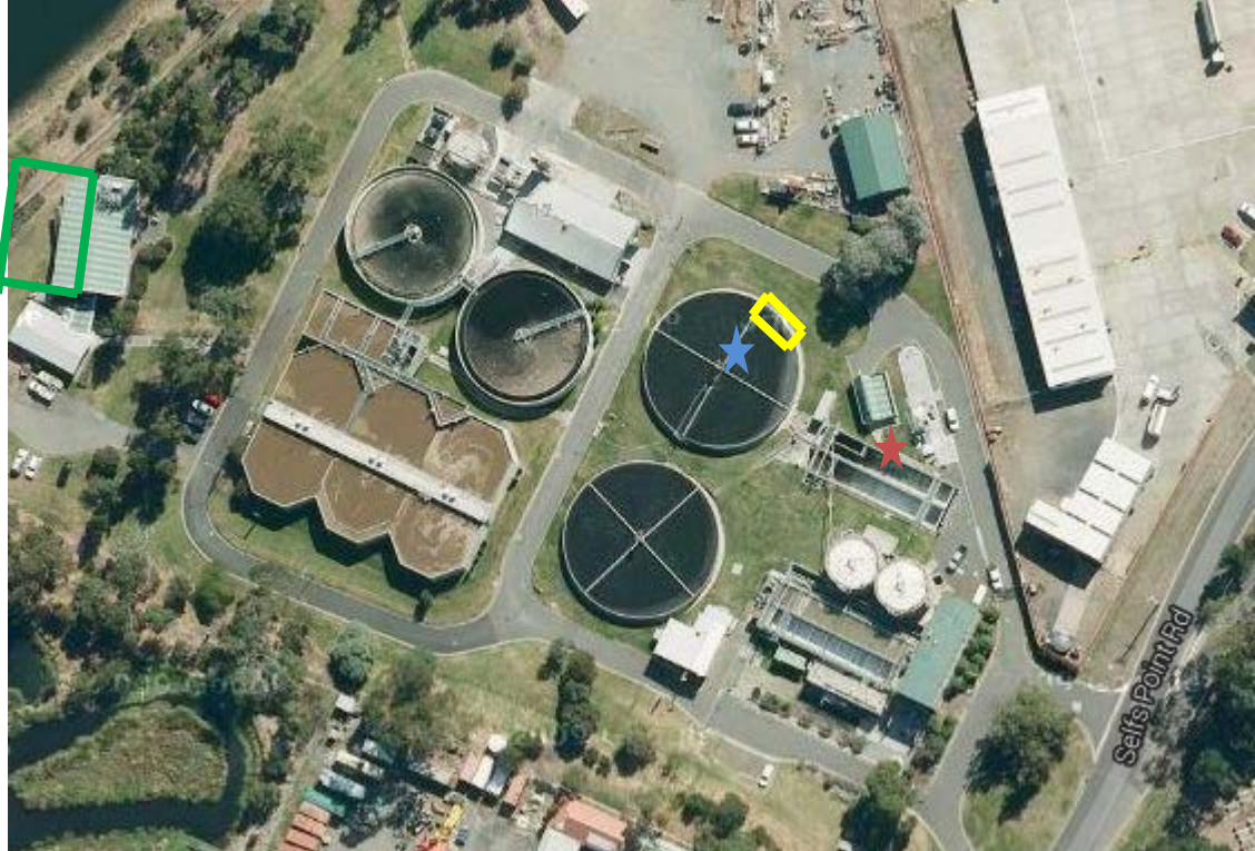
Google Map image of Self's Point Treatment Plant marking location of demonstration plant (yellow), the plant's feedwater source (red), the plant's discharge point (blue) and the TasWater laboratory (green)
