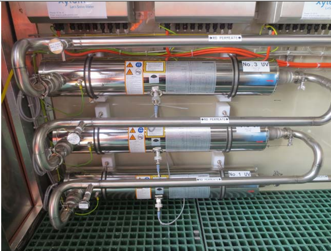
Figure x – UV reactors, UV, Section 3
