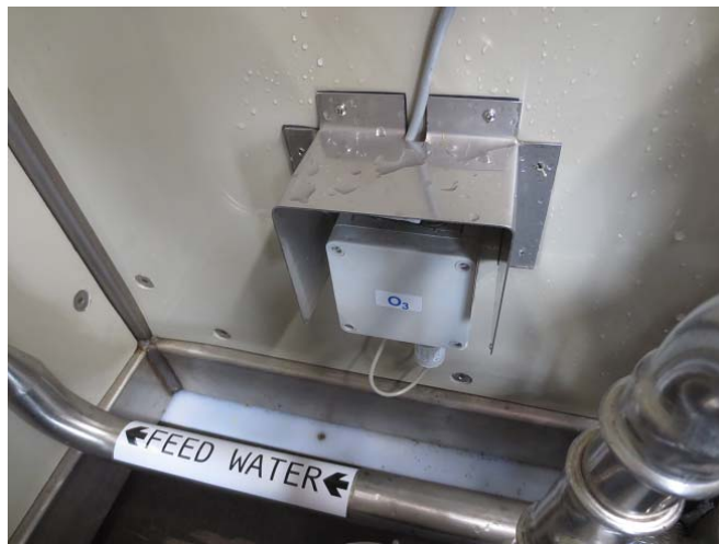
Figure x – Atmospheric ozone detector, Ozonation system, Section 1
