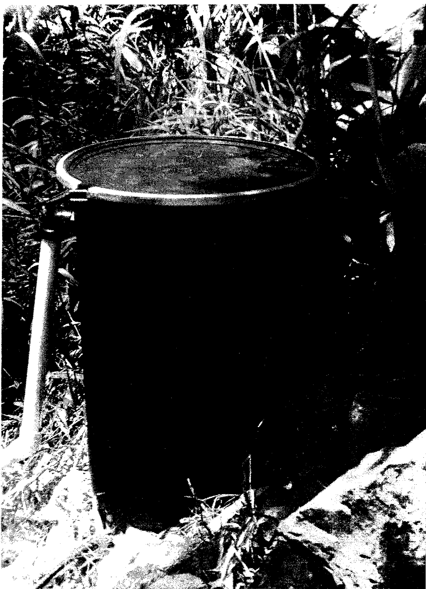
Figure 10.1 - Photo of a Typical Surge Tank in use in the USA
