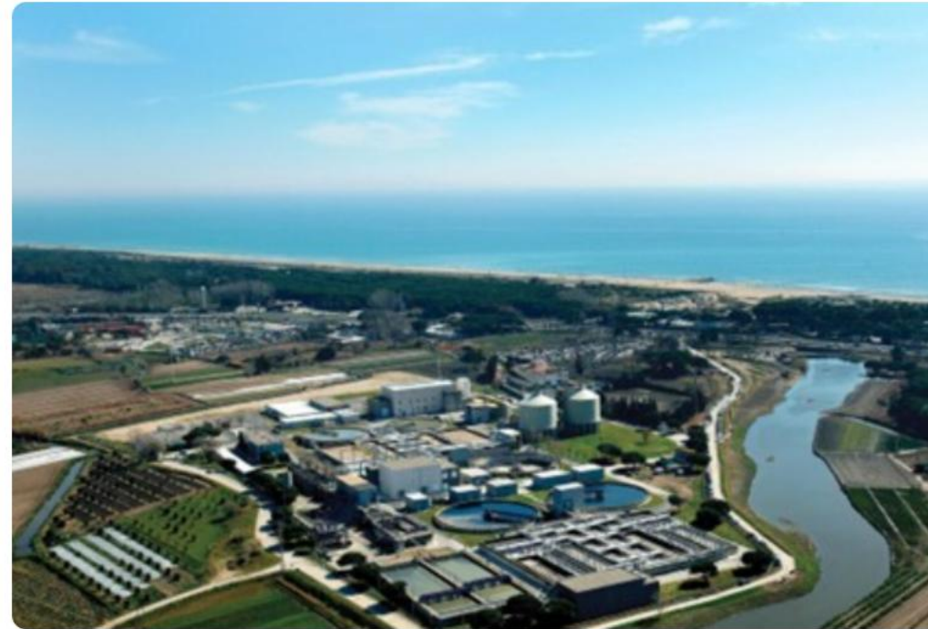
Aigües de Barcelona, Catalonia, Spain – building a demonstration plant to explore direct potable reuse in future
