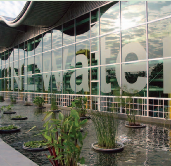
The Visitors' Centre at Singapore's NEWater reclamation plant.
